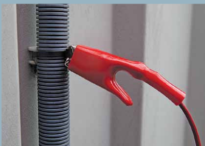
Small diameter cable tracing techniques
